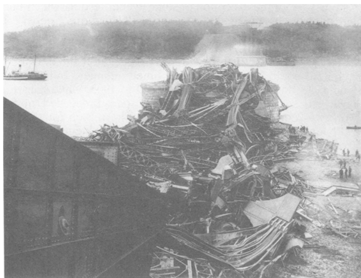
FIG. 2. Quebec Bridge: Aftermath of Collapse (Photo Courtesy Smithsonian Institution, National Museum of American History)
